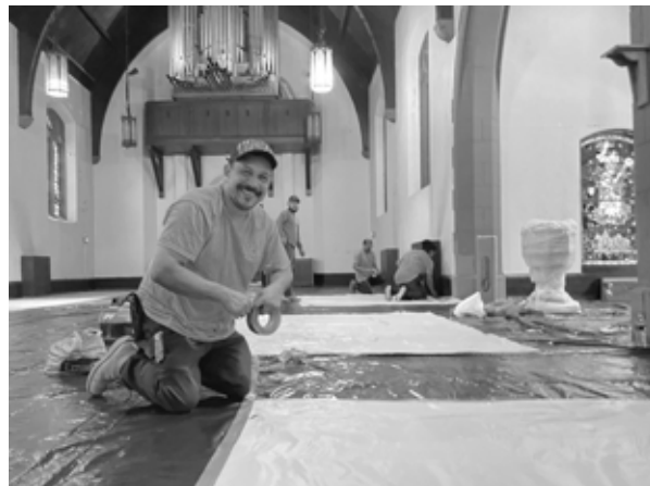
Floor protection was installed this week.
